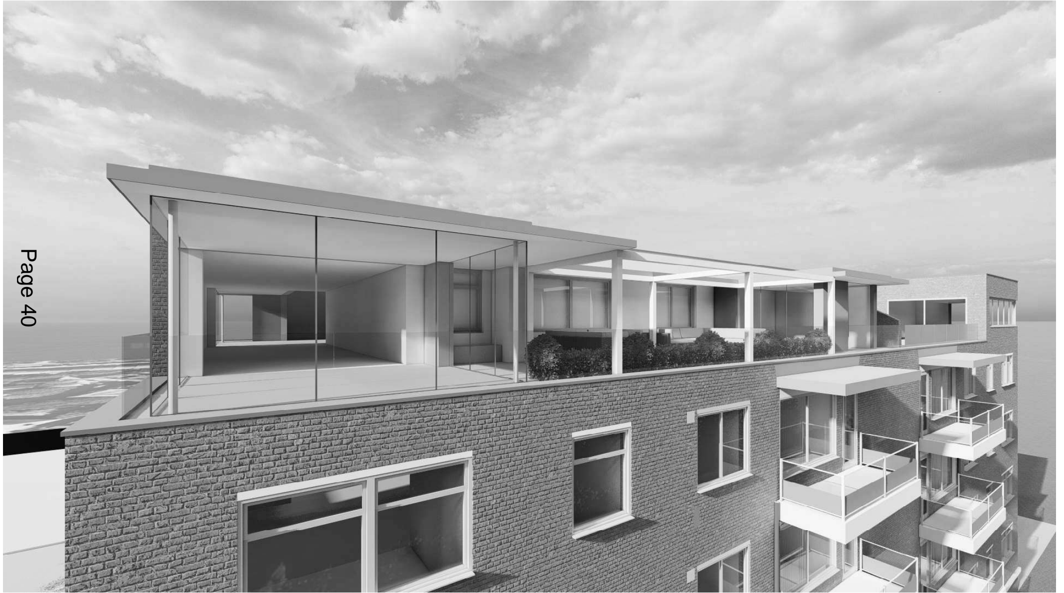
IMAGE 5: Proposed terrace level perspective to the rear of the property to illustrate the inset terrace, pergola and massing either end of the terrace
